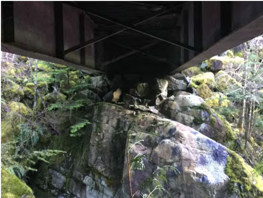
Left Bank Abutment when facing downstream
