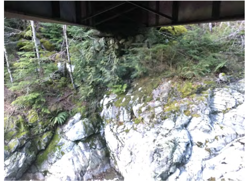
Right Bank Abutment when facing downstream
